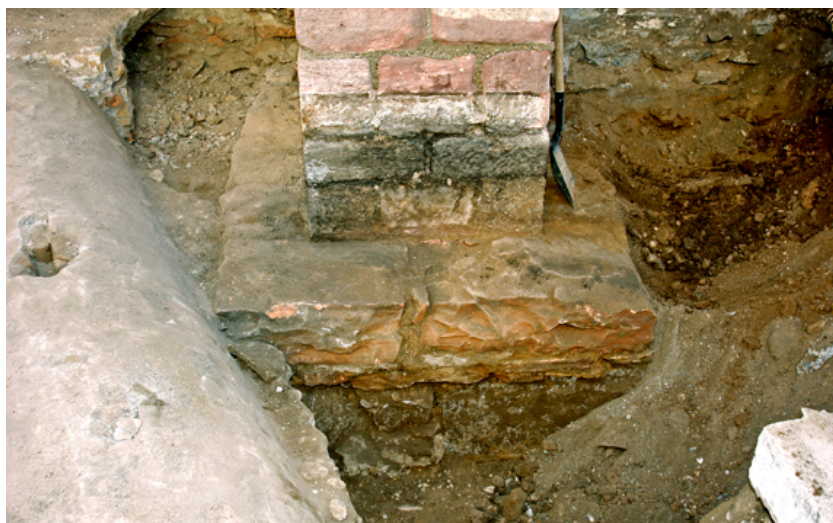
FIGURE 2. A stone pier footing. Photograph by Arnold Angle taken during the 2006 seismic upgrade.
