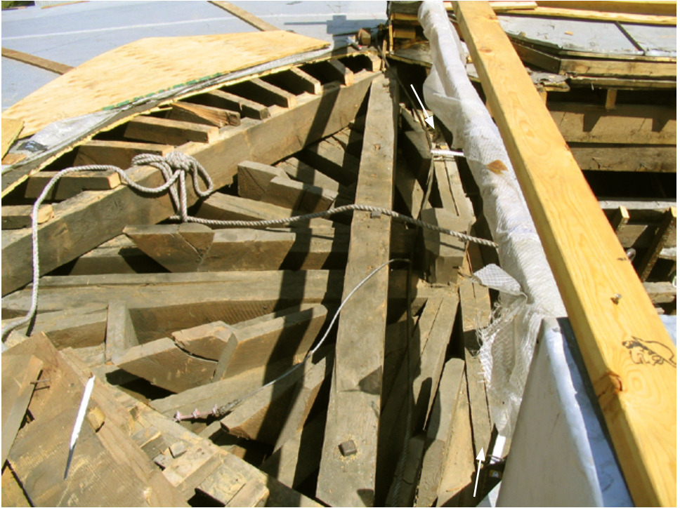
FIGURE 4. Trusses seen from the top of the Tabernacle, with the roof sheathing removed during the 2006 seismic upgrade. Here the half arches (radiating to the left in the photo) and the king arch intersect. Note how the top chord of the king arch (marked by arrows) bows five inches to the right, toward the center of the building, the result of 140 years of stress. A temporary safety railing and tarp are in the right of the photograph. Photo by Elwin C. Robison.
