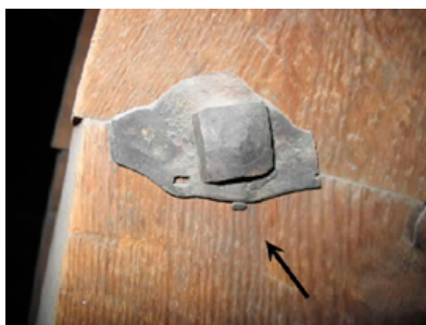
FIGURE 8 (top). A butt connection in one of the chords of the wood lattice-truss arches showing the half-inch-diameter wood pegs (black arrows), a hole drilled but missing a bolt (white arrow), a rawhide strip to control splitting, a new steel strap to supplement the rawhide, and a square bolt with a washer.
