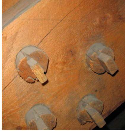
FIGURE 10. A pegged connection showing the wedges driven into the pegs perpendicular to the grain. Photo by Elwin C. Robison.
