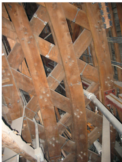
FIGURE 5. Wooden lattice truss arches of the Tabernacle. Note the new steel members, fire sprinkler piping to the right, and new steel strapping to prevent splitting of wood planks. Photo by Elwin C. Robison.
