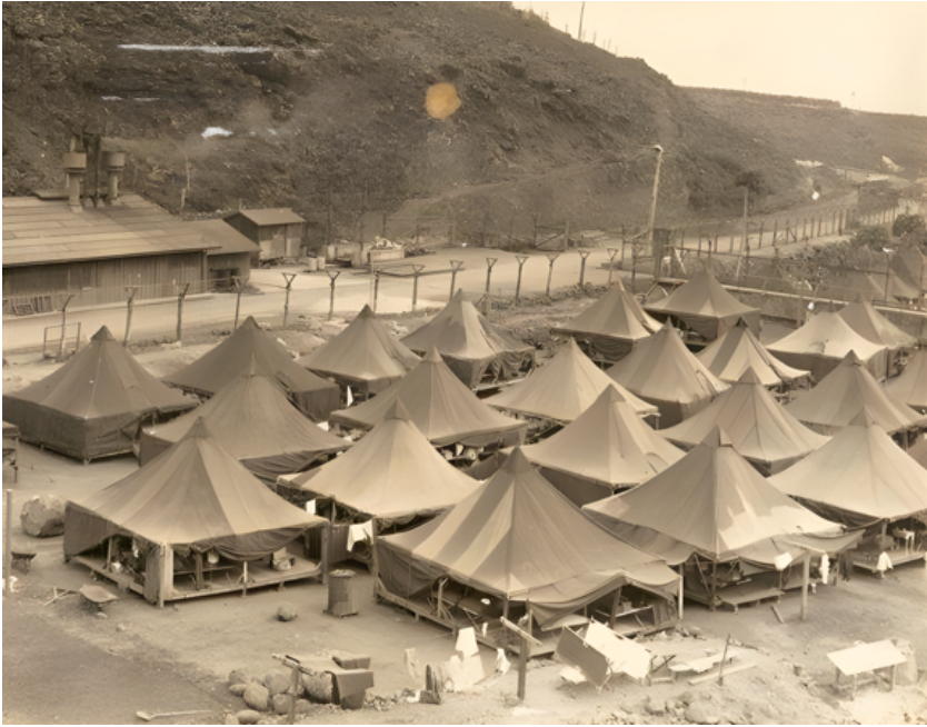
FIGURE 2. A view of the Honouliuli Concentration Camp in Hawai‘i. National Park Service.
